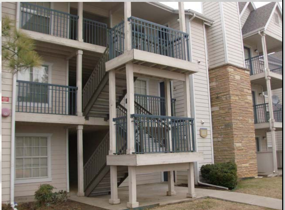
Pictured: Closed Riser Stair Treads at University Housing Complex.
