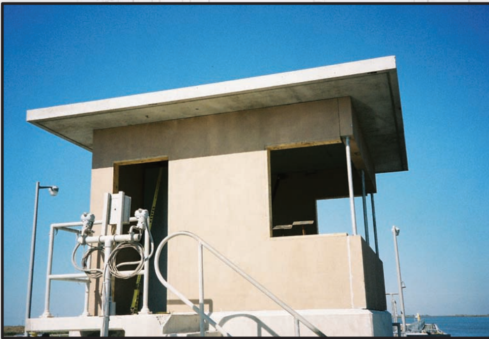
Century's precast concrete control room installed on the Intracoastal Waterway in Louisiana by the U. S. Army Corp of Engineers.
