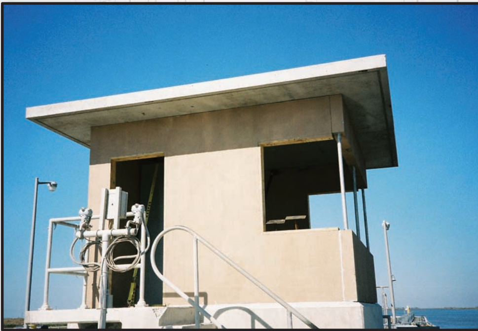
Century's precast concrete control room installed on the Intracoastal Waterway in Louisiana by the U. S. Army Corp of Engineers.
