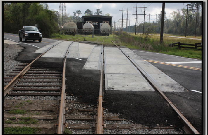
Century Concrete Railroad Crossings at Rail Car Repair Facility
