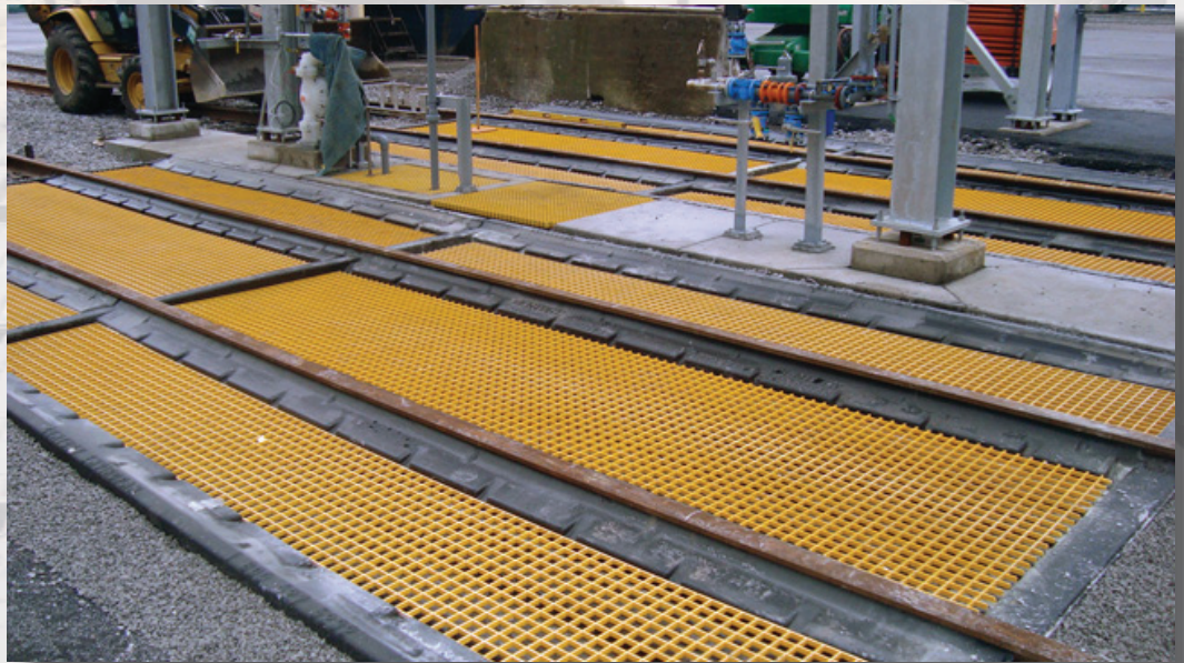
Century's HDPE railroad spill collection pans at petrochemical railroad tank car loading rack.
