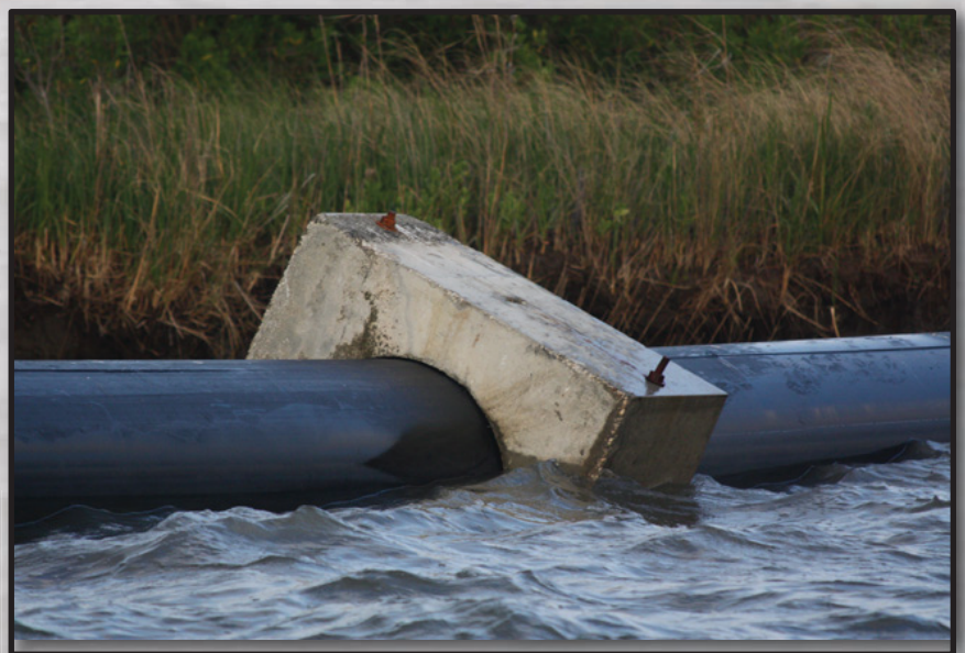
Century Precast Concrete Pipe Weight on Dredge Spoil Discharge Pipe
