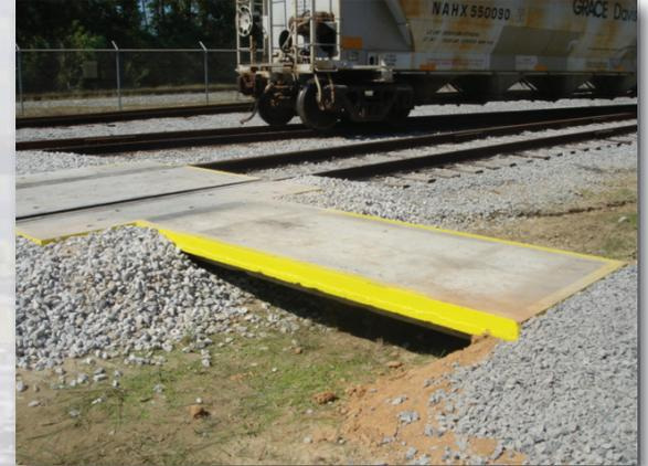
*Century Group Inc's precast concrete pedestrian crosswalk installed in an industrial railroad spur.*
