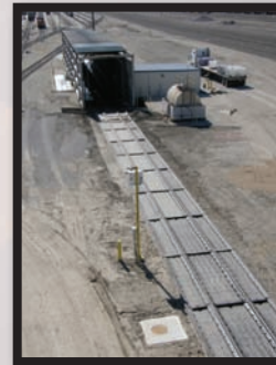
Century HDPE Railcar Spill Containment Pans at Class I Railroad Maintenance Yard
