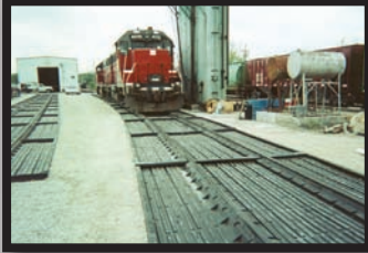
Shortline Railroad Fueling & Maintenance Facility
