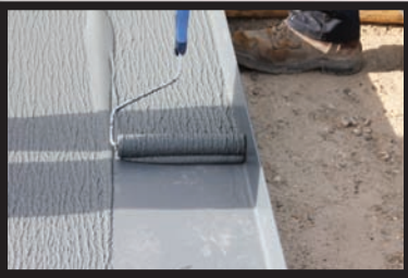
Textured coating being applied to Century Group's steel railroad spill containment pans.
