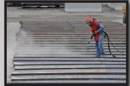
Century Group team member blasting steel spill collection pans.
