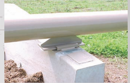
Concrete Pipe Support with Pipe Restraint/Expansion Bracket
