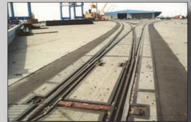
Turnout Concrete Crossing Container Port
