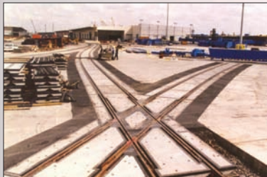
Diamond Concrete Grade Crossing
