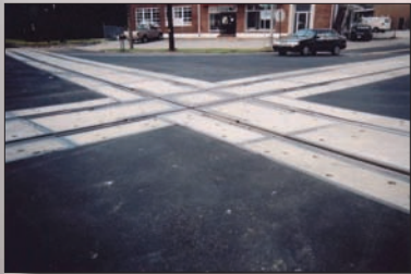
Diamond Concrete Grade Crossing on Shortline Railroad
